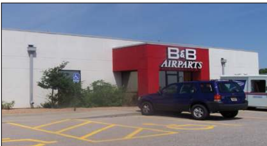
B&B Airparts facility, Wichita, KS.
